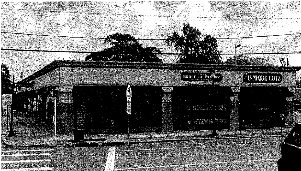
543 Merrick Road, Lynbrook
