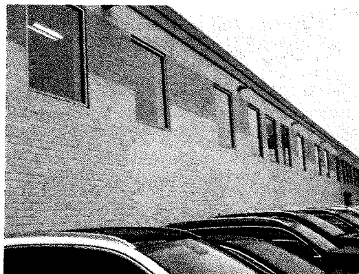
View of entire side wall that has been repeatedly patched
