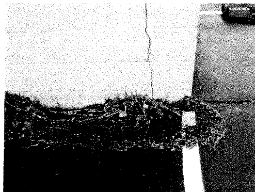
(Exterior) wall with apparent structural crack
