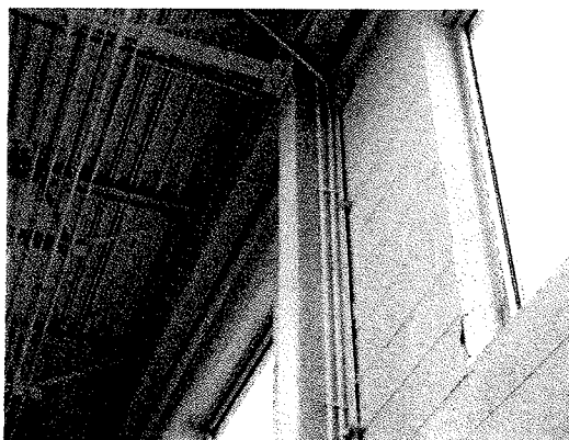
Interior wall with atypical construction of steel beams along exterior wall supporting ceiling and structure — also note cracking and damage at window
