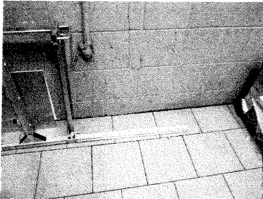
Rear corner/inside with water pouring through crack in wall and up from floor Interior floor water damage
